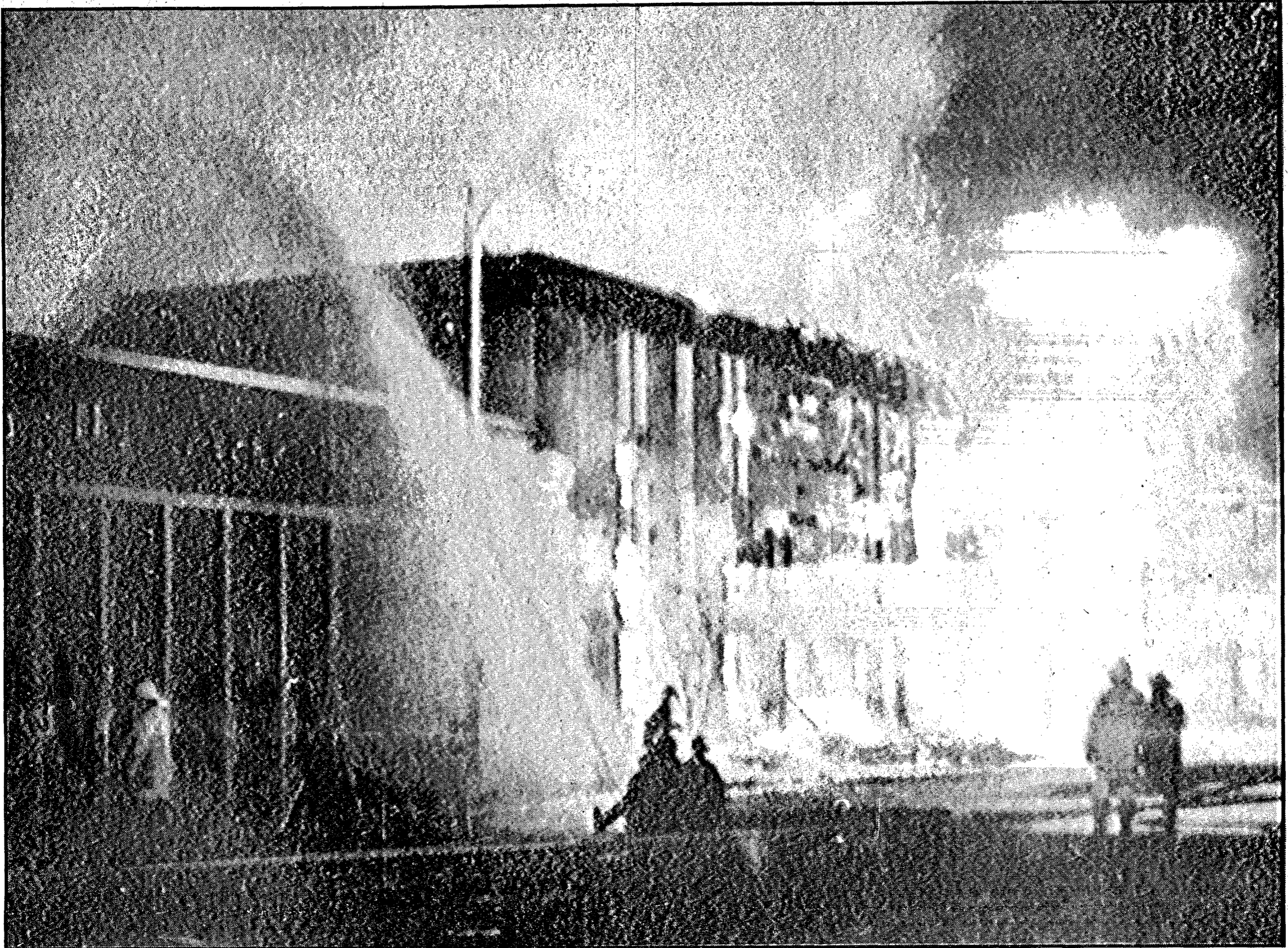
FLAMES SHOOT THROUGH the roof of the State National Bank and Trust Co. in the wee hours of the morning Thursday. Fire fighters pour water onto the bank building and the adjoining Wayne Herald office. A fire wall between the two buildings, along with the efforts of firemen, prevented flames from spreading to the newspaper building. The bank was gutted and several other adjoining businesses were destroyed in the blaze.
